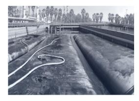
The operation was a success and CTP ambiente was able to rise to certain challenges: in effect, the sludge was far from uniform and contained a large quantity of waste, with storms broadly filling the tank. Despite unpredictable pumping, due to a combination of these two factors, 42 000 m³ (54 950 yd³) were extracted in 1,5 months. In the end, 2600 m³ (3400 yd³) of sludge was stored in the geotextile membranes, leaving 955 tons of dry matter to be disposed of by a specialist facility.
